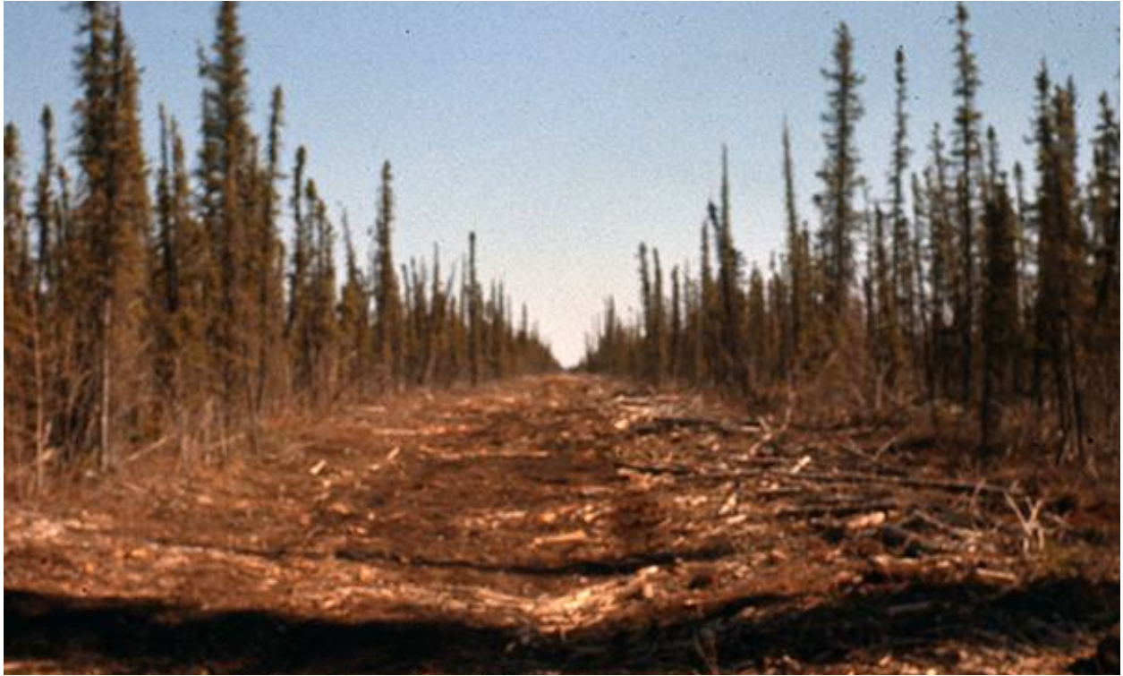
Fig. 3.6: Mackenzie Highway slash road north of Norman Wells, May 1974. N-2011-004: 0094, David Sherstone collection, NWT Archives, Canada. Although the highway never made it as far as Norman Wells, slash crews often worked well ahead of gravelling teams further south. Hire North workers regularly outpaced heavy equipment operators by a considerable margin. Environmental regulations requiring additional permitting in ecologically sensitive areas also encouraged clearing teams to work ahead in areas already approved for construction.
